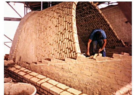
Bricklaying a nubian dome without supporting form
