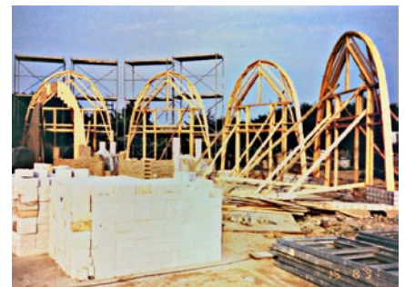
Forms for the nubian vaults
