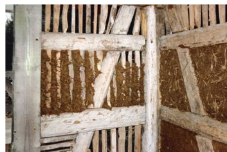
Repairing the timber-frame infill panels
