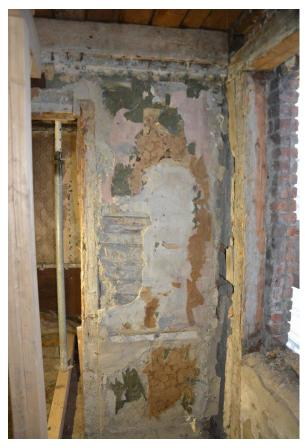
03 Traditional type of vernacular Nordic timber and earth construction (earth mortar layer between squared timber in wood framing) with "rapping" (a type of Norwegian clay plaster on wooden surfaces), in the house Smedbakken 5 from 1845/46 in Trondheim, Norway (source: author)
