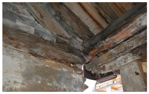
02 Enormous structural damage to all of the geometric envelopes of the 175-year-old residential house at Smedbakken 5 about 40 years after the micro-meteorological reversal of the vapour permeability and the dew point. (Source: Author)
