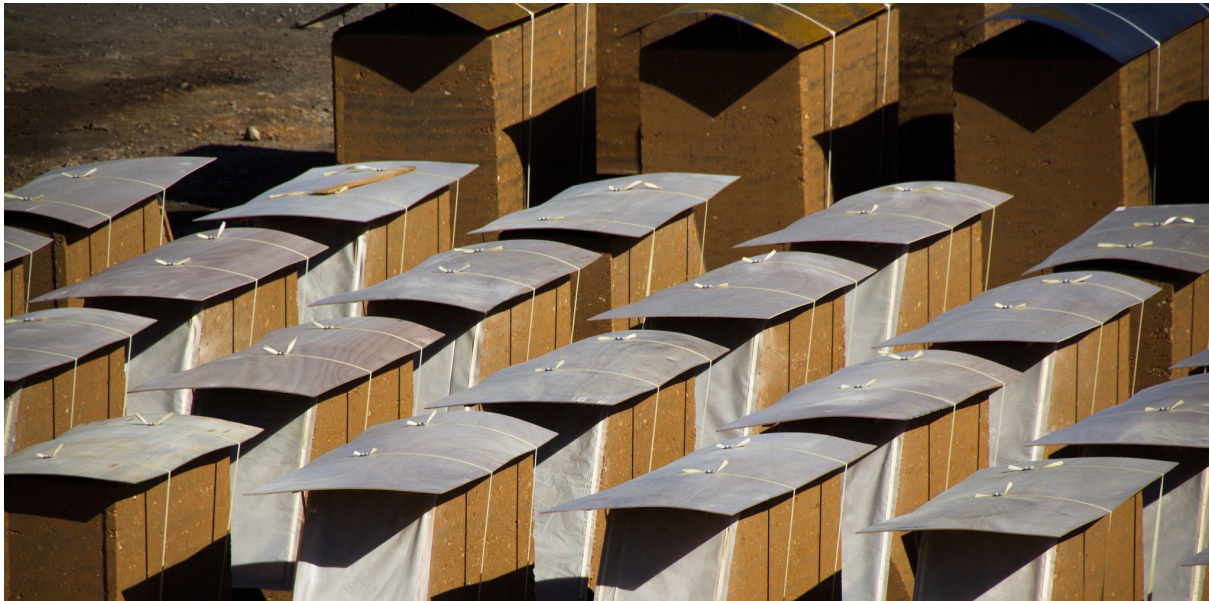
09 Storage and drying of the earth blocks (© M. Valcarce)
