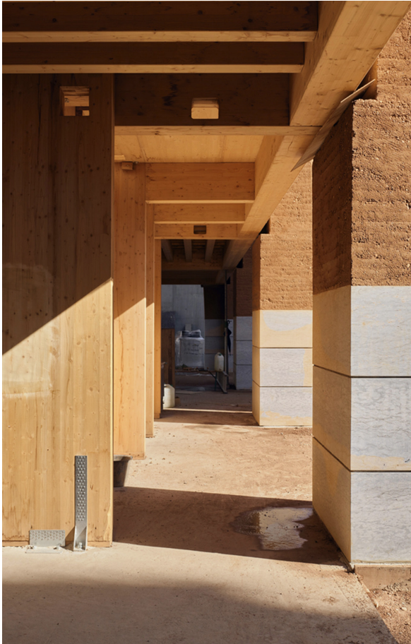
06 Three materials: wood, stone and rammed earth (© F. Fouillet)
