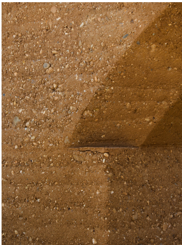
10 Prototype of the arch chamfer (© M. Valcarce)
