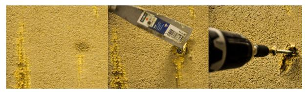
04 Sequence of the dismantling process of earth dry lining boards
